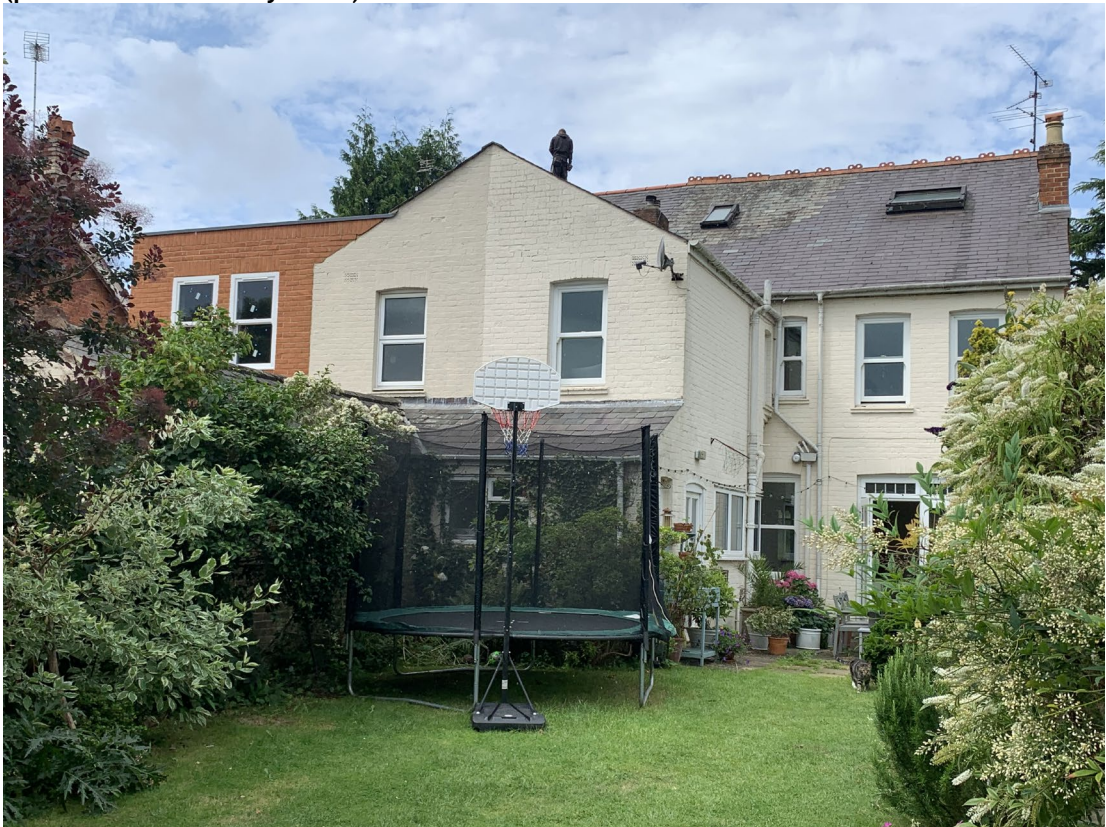
Photo 1: Existing rear elevation with part of rear extension at 80 Albert Road (photo taken 28 th July 2021)
